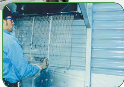
Inlet strainer inspection for Series 3000
