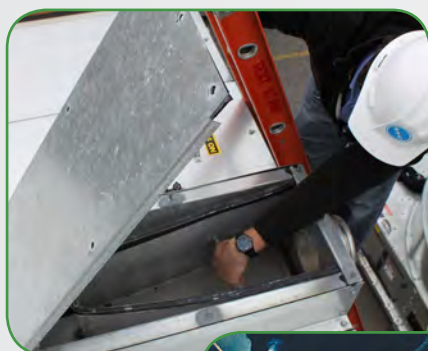
Inlet strainer inspection for Series 1500
